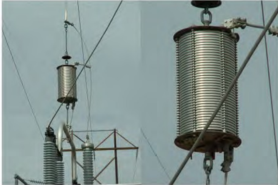
Figure 5.16: Wave Trap
