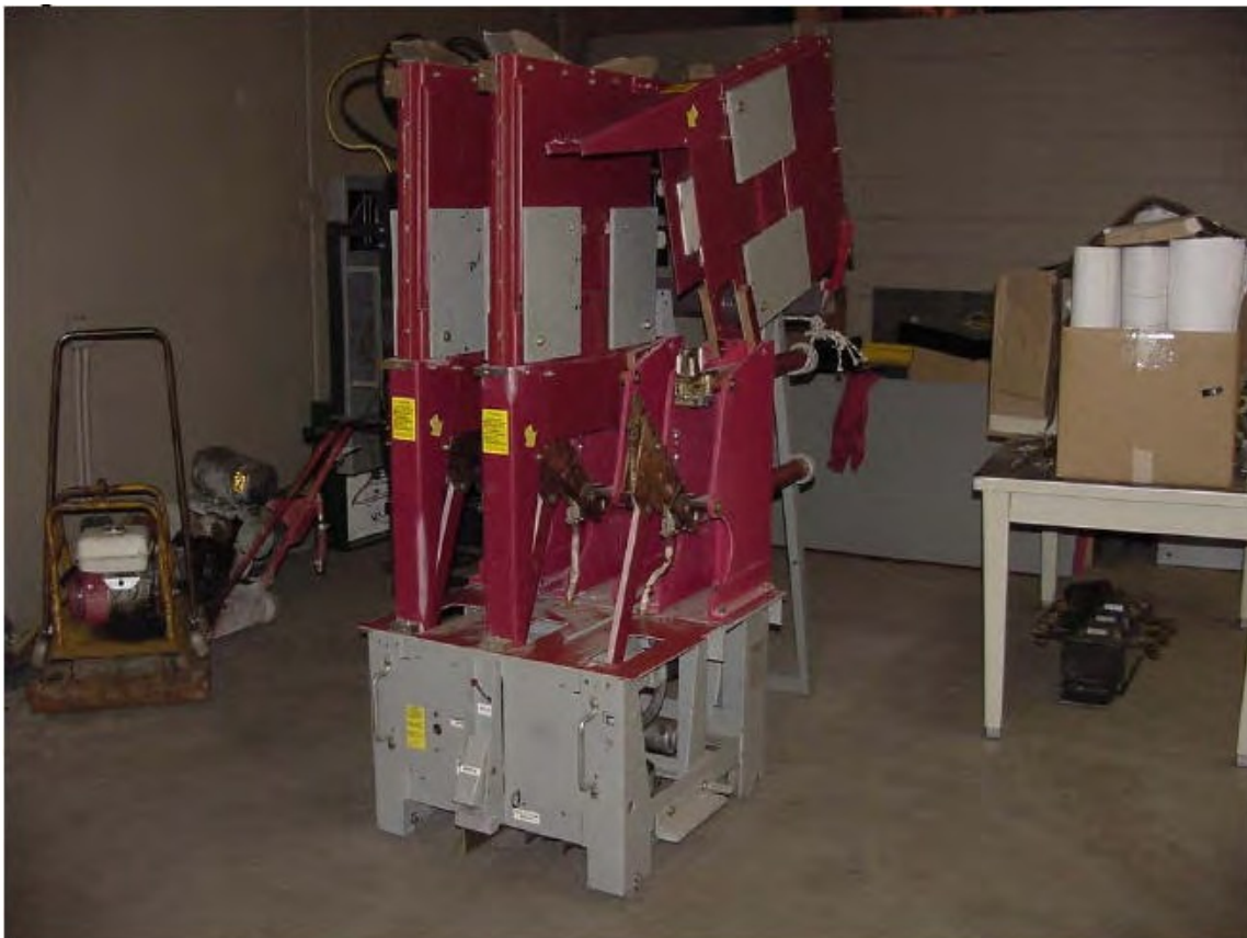
Figure 5.3: Air Circuit Breaker
