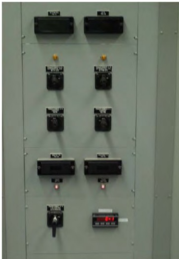
Figure 5.16b: Bottom half of Transformer Relay Panel
